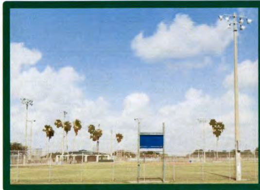
Harlingen Sporting Complex HID lighting
