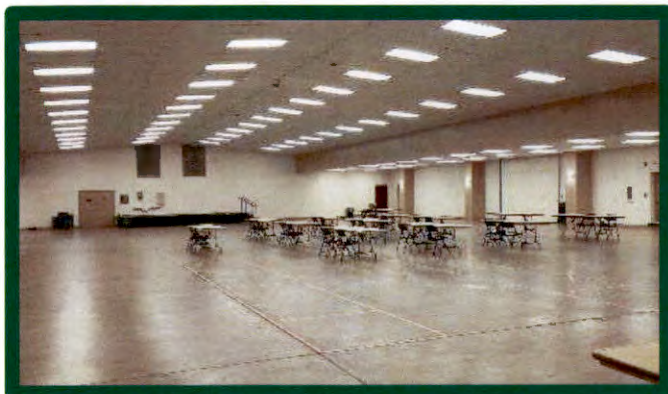
Casa De Amistad inefficient fluorescent lighting
