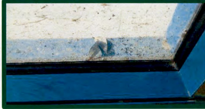
Single-pane windows at the Harlingen Public Library
