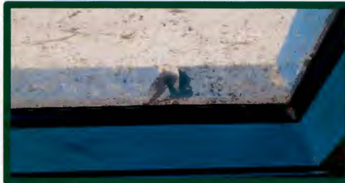
Single-pane windows at the Harlingen Public Library
