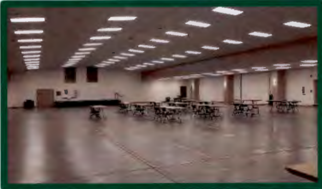
Casa De Amistad inefficient fluorescent lighting
