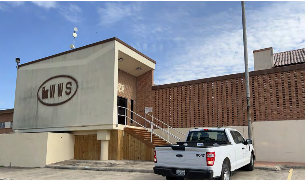
Harlingen Waterworks System Water Filtration Plant, 2024
