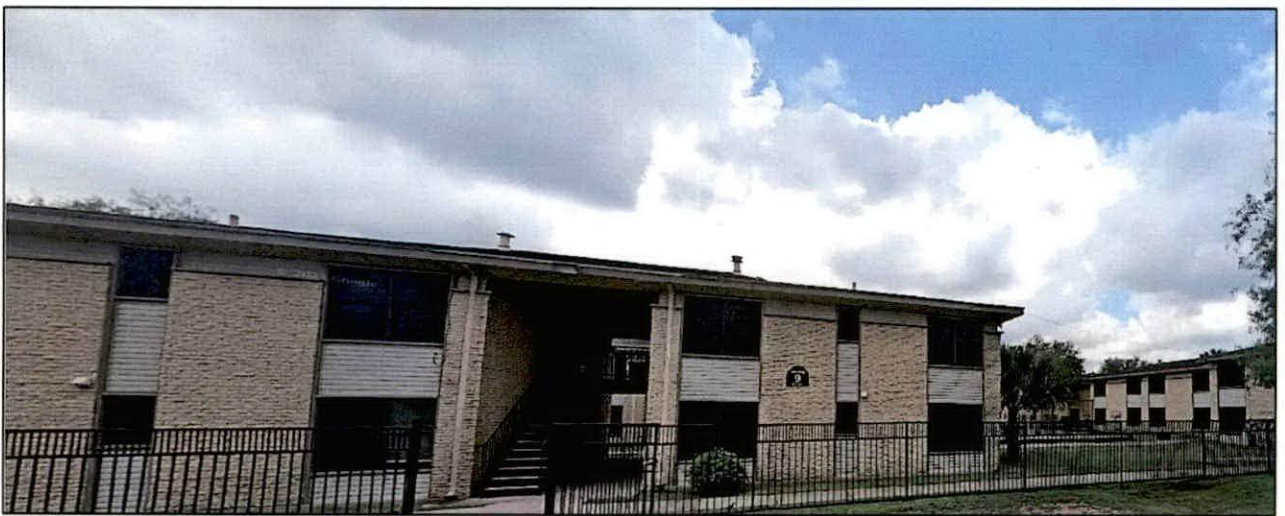
Figure 2. Photo of existing building on site
