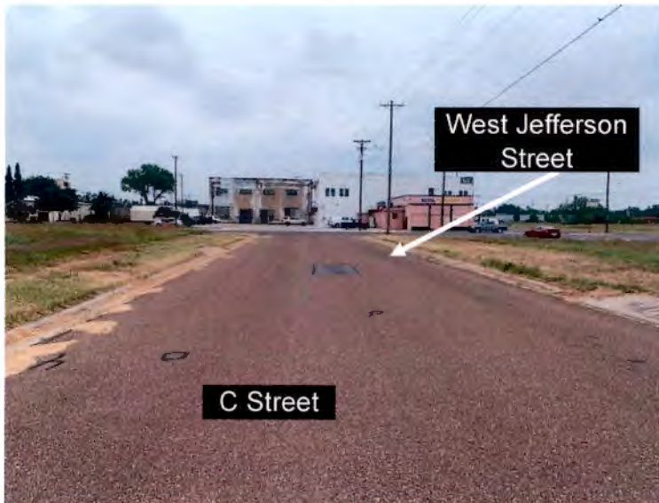
Figure 5 - C Street View to the South
