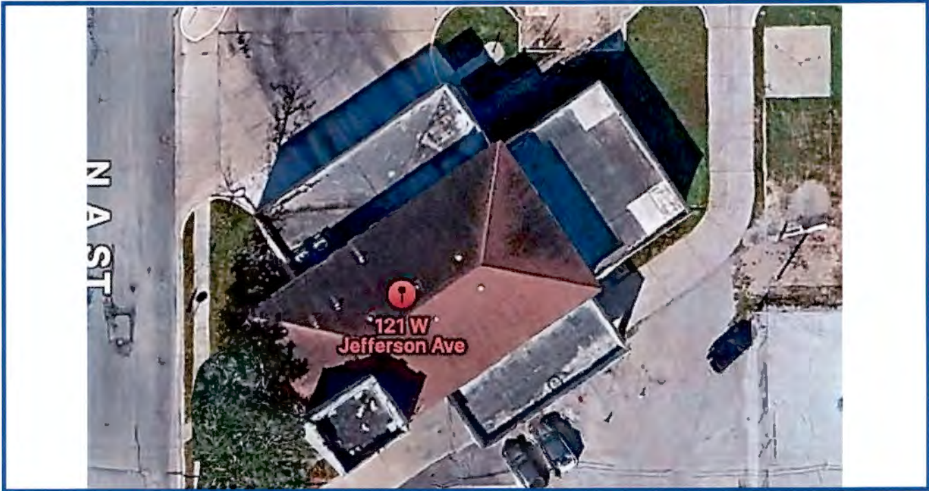
Approximate Roof Area: 4,300 square feet
