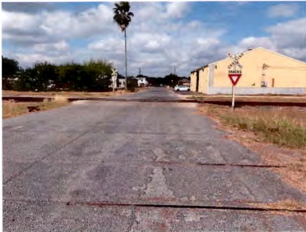
Second Street - Northbound
