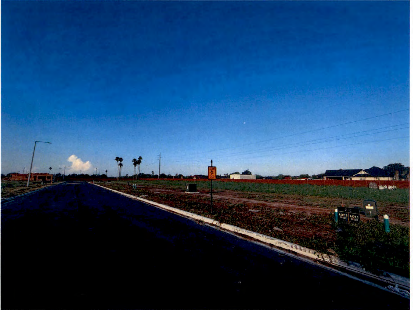
Street View from James Street
