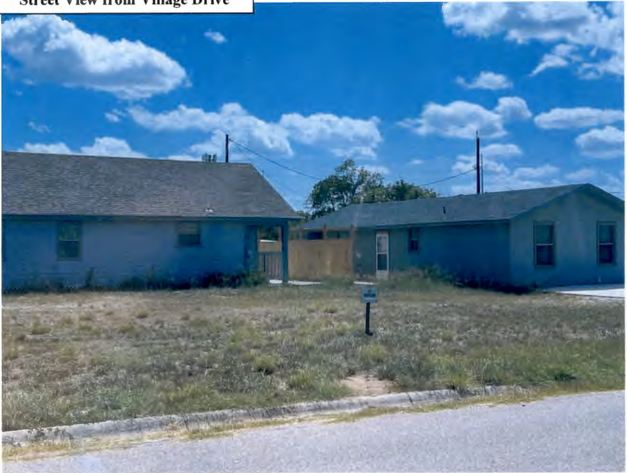
Street View from Village Drive
