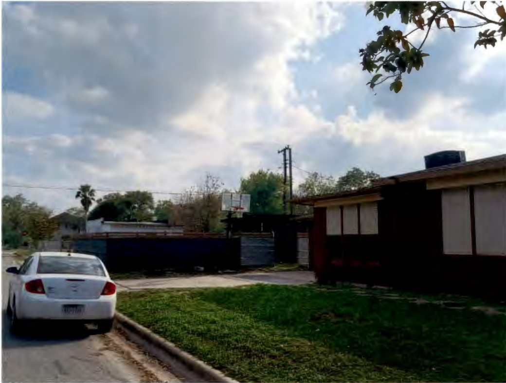
Street View from South “B” Street
