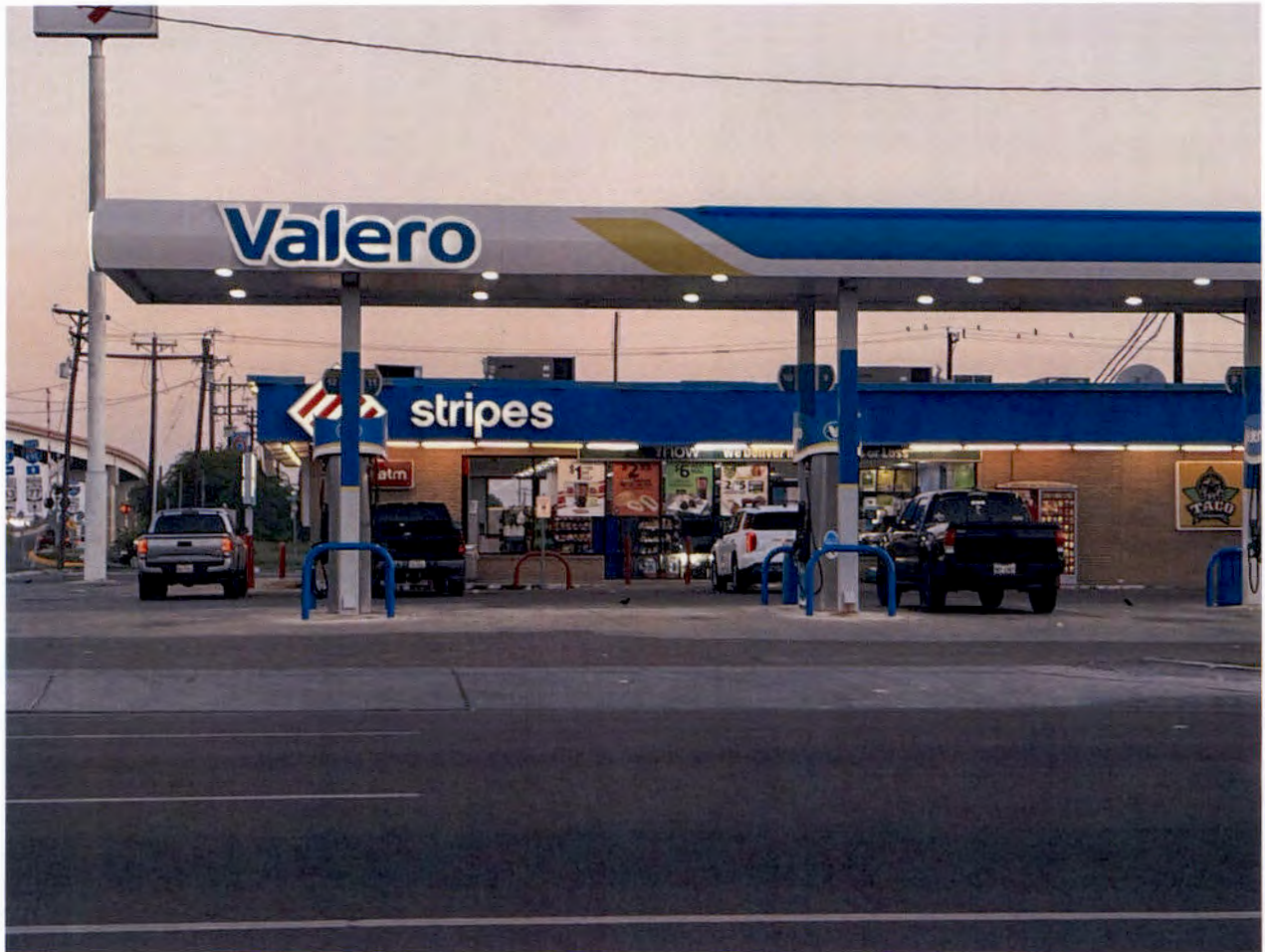
Street View from West Tyler
