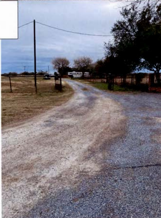
View of the private roadway leading to the proposed subdivision
